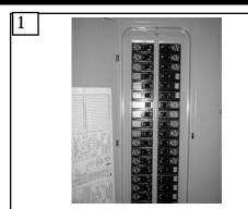
Before you begin installing the fan, Switch power off at Service panel and lock service disconnecting means to prevent power from being switched on accidentally. When the service disconnecting means cannot be locked, securely fasten a prominent warning device, such as a tag, to the service panel.
